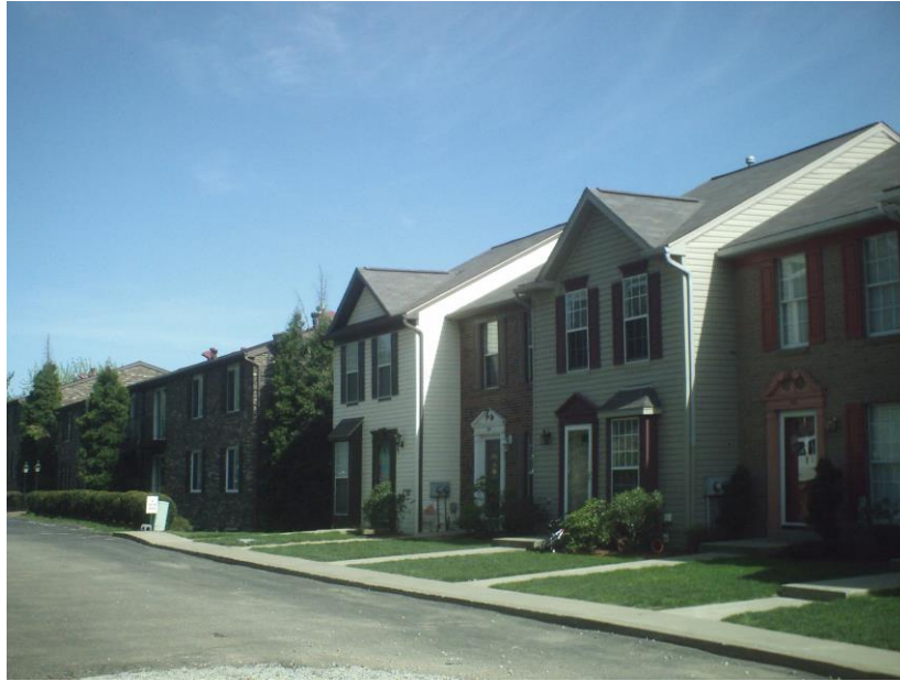
Well-maintained housing units. Source: Remington, Vernick & Beach Engineers
